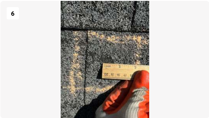
Close view of Hail Impact measuring about 1/2 inch diameter NOT from August 18th, 2024 Hail Storm.
