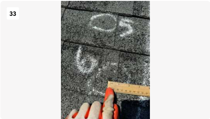
Front C5 and C6 1/4 inch Hail Impact Close Up
