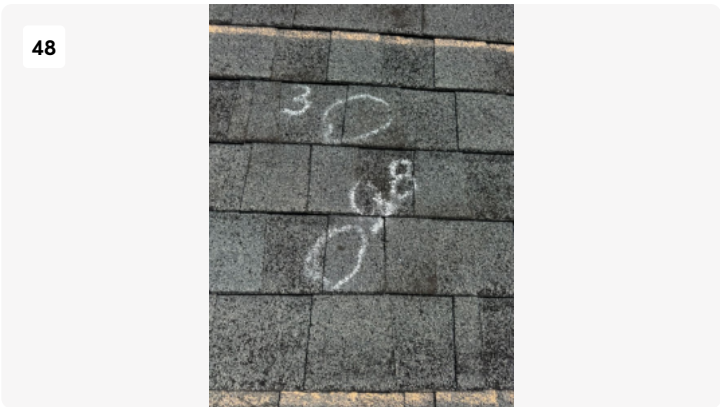
Left C7 and C8 1/4 inch Hail Impact Close Up
