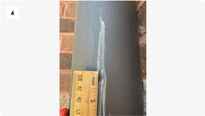
1/4 inch Hail Impact to Downspout
