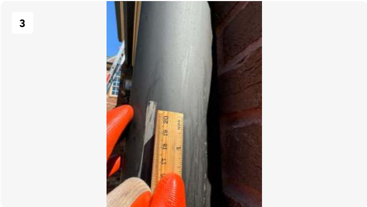
1/4 inch Hail Impact to Downspout
