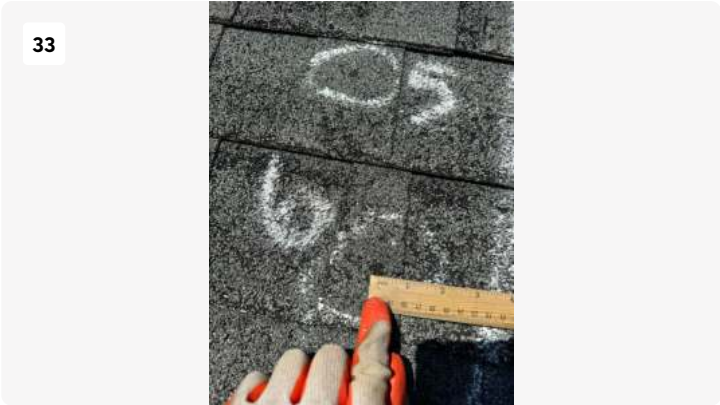
Front C5 and C6 1/4 inch Hail Impact Close Up
