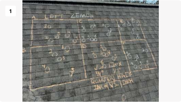
Left Facet 1/4 inch Hail Impacts Correlating with the August 18th, 2024 Hail Storm
