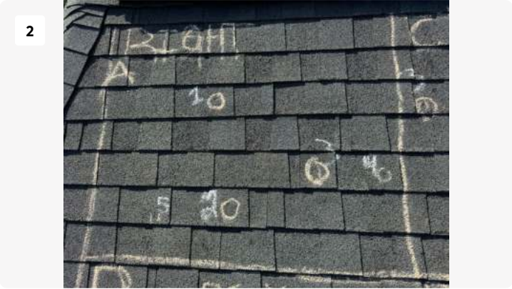
Right Facet - Section "A" 1/4 inch Hail Impacts
