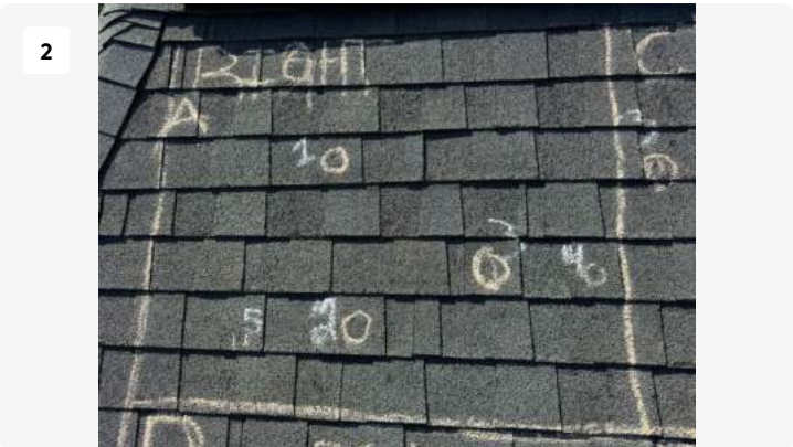
Right Facet - Section "A" 1/4 inch Hail Impacts
