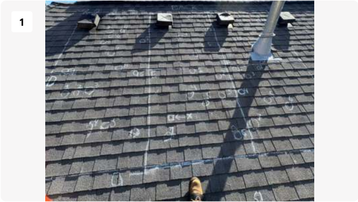
Back Facet 1/4 inch Hail Impacts Correlating with the August 18th, 2024 Hail Storm
