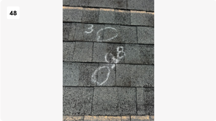
Left C7 and C8 1/4 inch Hail Impact Close Up
