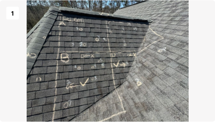
Right Facet 1/4 inch Hail Impacts Correlating with the August 18th, 2024 Hail Storm
