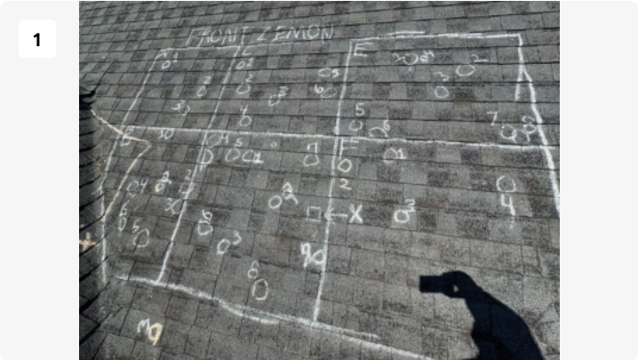
Front Facet 1/4 inch Hail Impacts Correlating with the August 18th, 2024 Hail Storm
