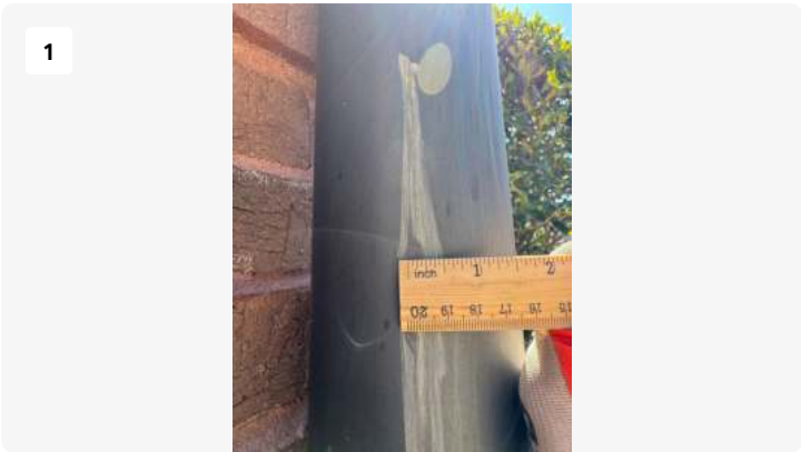
1/4 inch Hail Impact to Downspout
