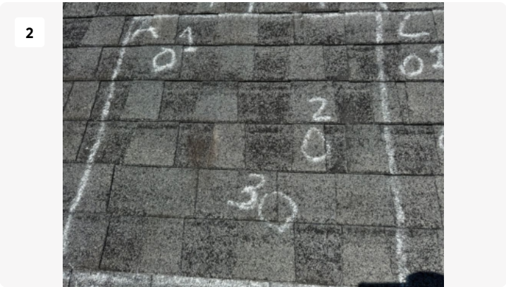
Front Facet - Section "A" 1/4 inch Hail Impacts
