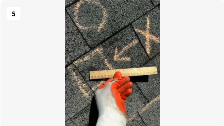
Hail Impact measuring about 1/2 inch diameter NOT from August 18th, 2024 Hail Storm.
