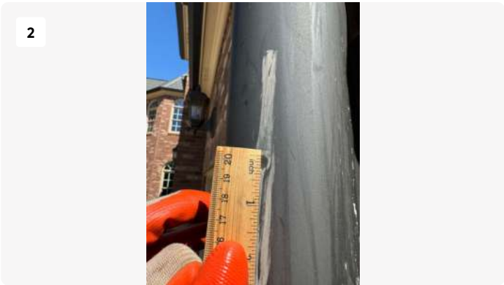
1/4 inch Hail Impact to Downspout
