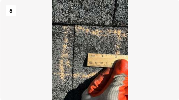
Close view of Hail Impact measuring about 1/2 inch diameter NOT from August 18th, 2024 Hail Storm.
